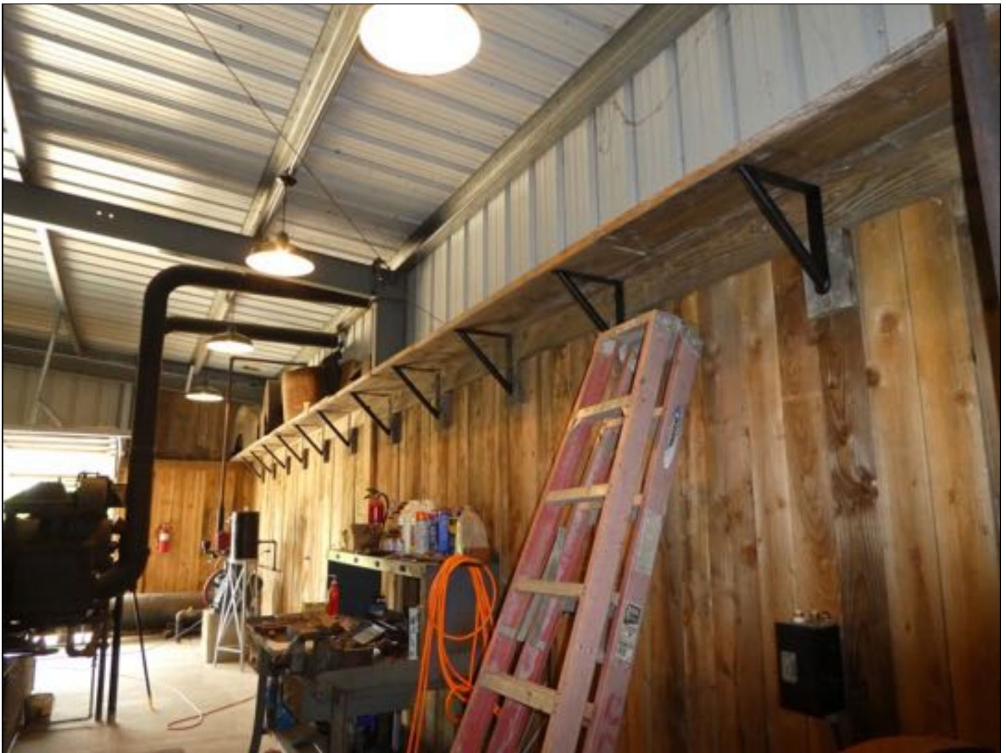
This photo shows some of the progress we have made on the building where the 200 Western engine is located in the Citrus Park in Riverside. We've installed paneling, with a display shelf above the paneling. More to follow.
