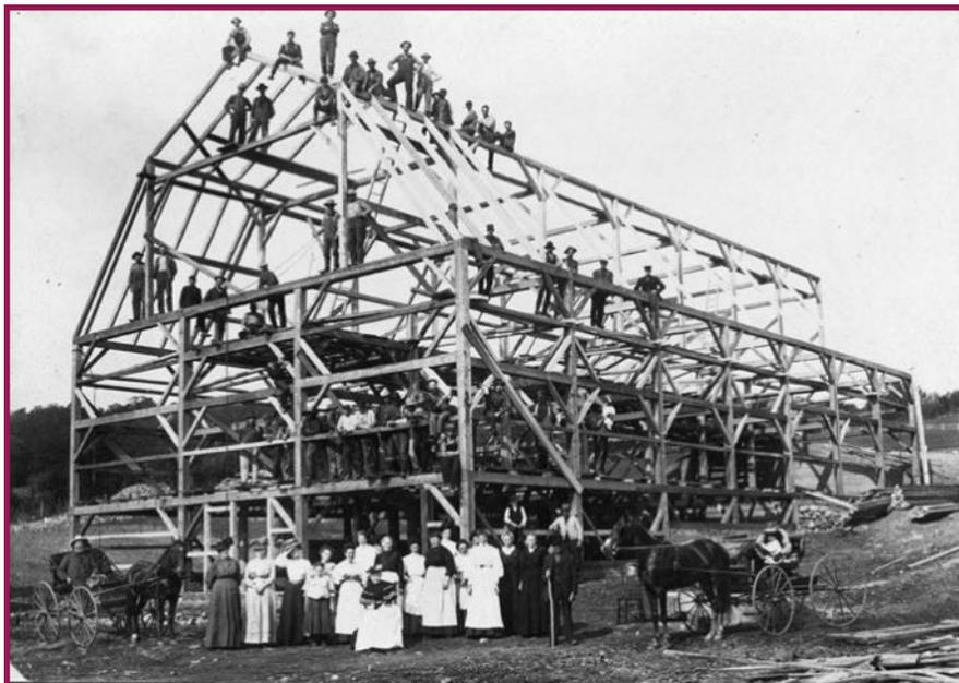
Ropes held by men kept the frame from tipping too far. After the parts were all tied together with the oak pins or the long bolts, the rafters were hoisted up and placed into position.
