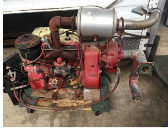
Here is a picture of the two cylinder Wisconsin that I am getting running for the Orange Empire Railway Museum. Operates a fire pump and is used to help with brush fires.
